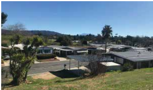
Hillcrest Mobile Estates; recently consolidated by South Mesa Water Company
