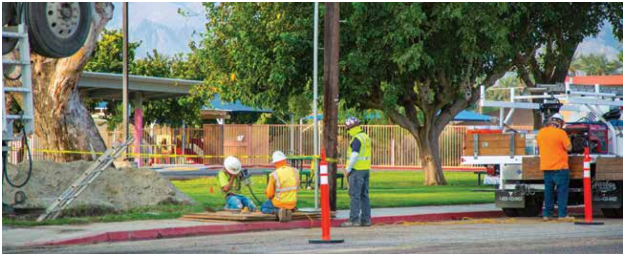
Workers conducting repairs.
